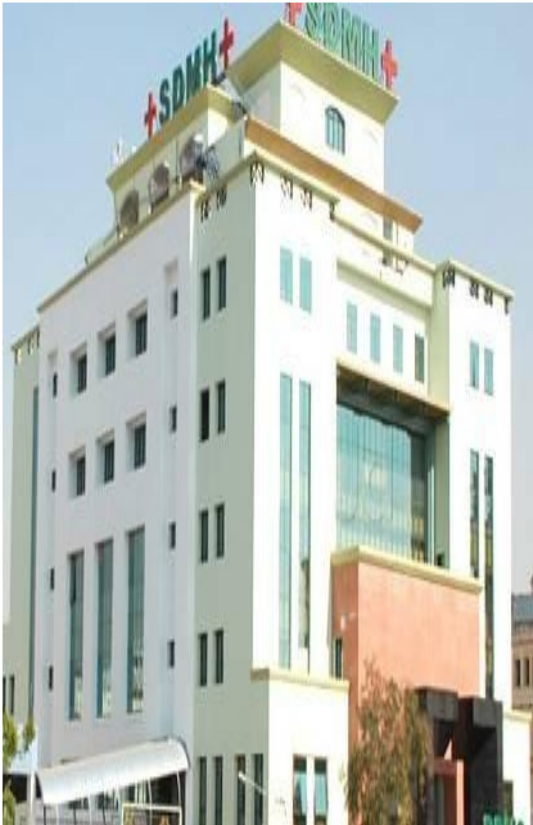
Figure 3.8: Santokba Durlabhji Memorial Hospital, Jaipur
