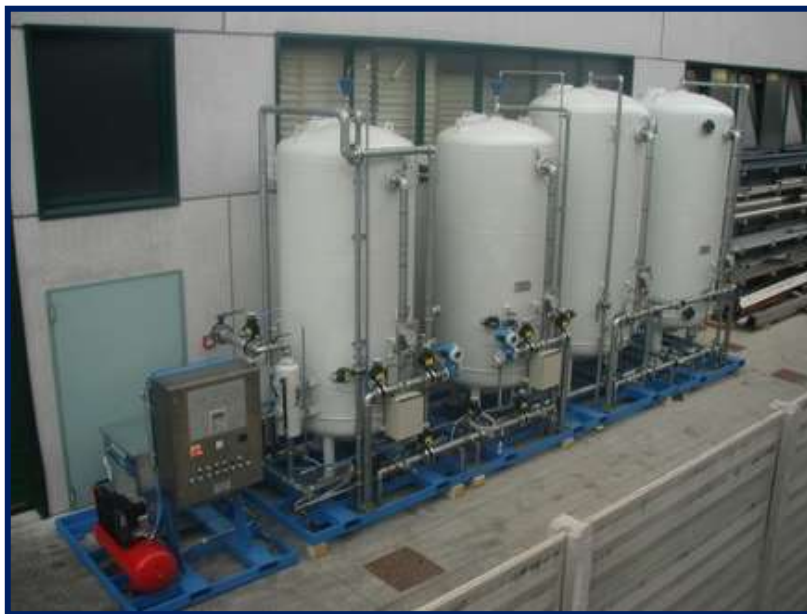
Figure 1.4: Biological Water Filtration
